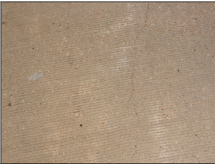
Typical longitudinal deck crack
