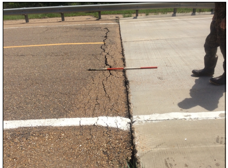
Abutment #2 roadway settlement
