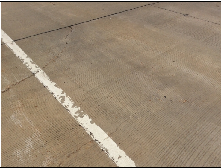
Abutment #1 approach slab cracks
