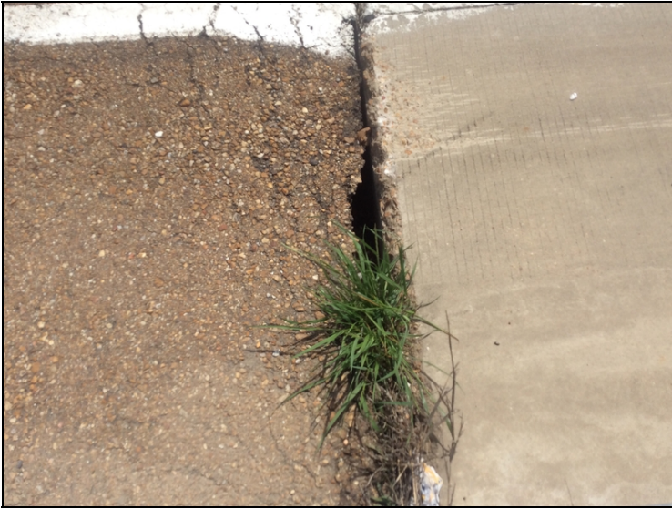
Abutment #2 open joint between roadway and approach slab
