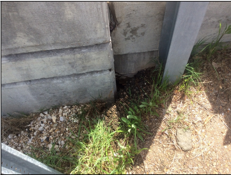
Minor erosion under approach slab abutment #1 left and right side
