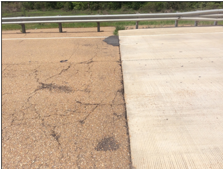
Abutment #1 joint at approach slab. And roadway settlement
